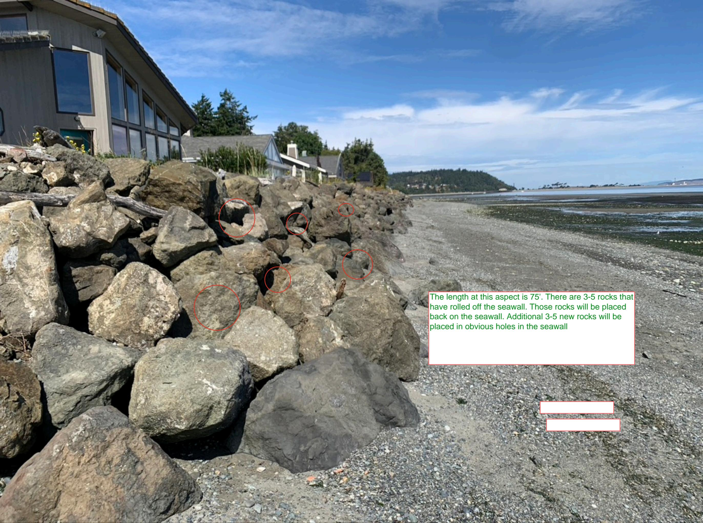
The length at this aspect is 75'. There are 3-5 rocks that have rolled off the seawall. Those rocks will be placed back on the seawall. Additional 3-5 new rocks will be placed in obvious holes in the seawall
