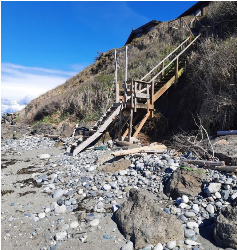
Figure 6. Erosion behind the pull-system stairs that provide access to the shoreline.
