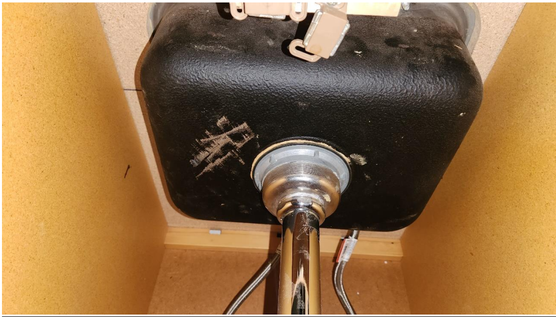
Sample #20. Black Sink Undercoating on 7 Sinks. (See the field report for locations.)
